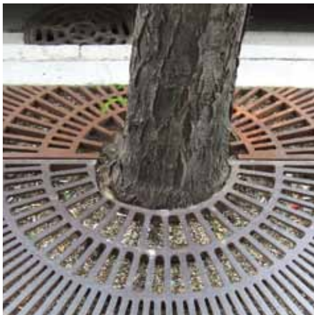
A 24" removable center ring is inserted to the grate to accomodates tree growth for a maturing tree.
