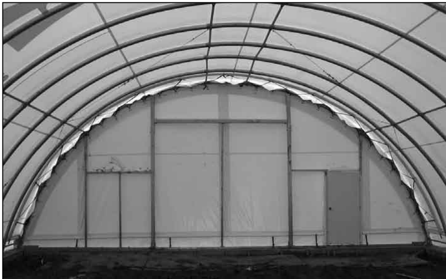
Photos show end panel examples. Lower photo shows an installed panel as seen from the inside.
